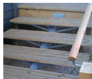
Q-Grip Strips fitted into Q-Deck
